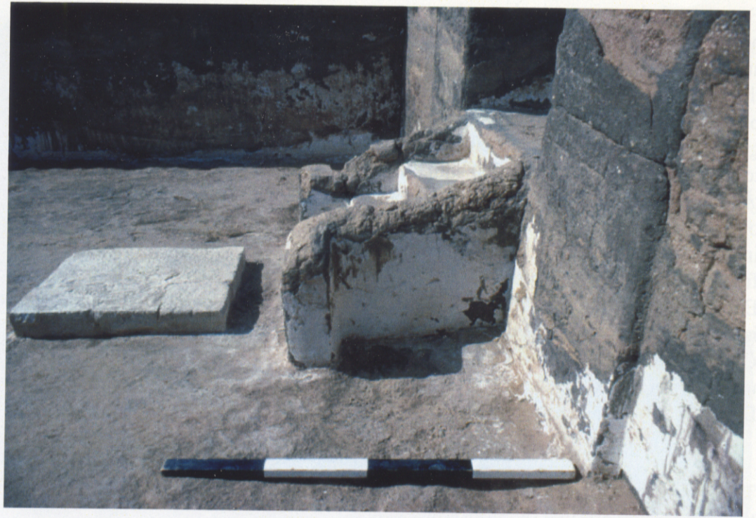
Inner Hall: View northwards across the Inner Hall, showing the stairs leading up to the Sanctuary, and a low limestone slab set in the floor, probably an offering-table
